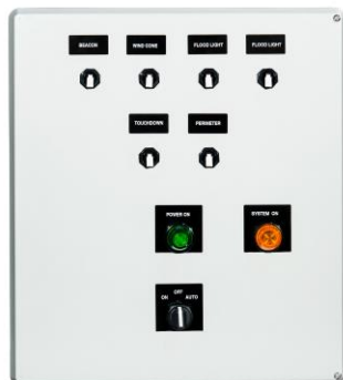
HELIPORT LIGHTING CONTROLLER PHC-61001-1-SC1
